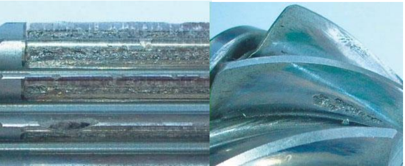
Pitting (common gear failure caused by surface damage from cyclic contact stress)
